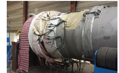
Heat treatment by local application
